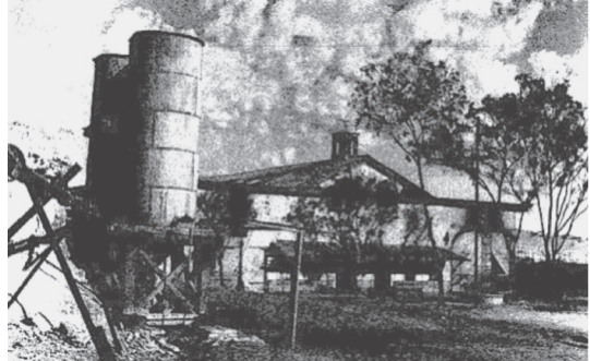
37b. Desalination device with a capacity of 34 m 3 /day built in 1851 in the port city of Caldera, mainly to power locomotive boilers (from: Gilliss J.M., 1855, p. 248).
